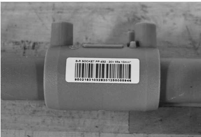
Figure F-18. Push in the electrofusion socket up to the marked position on the pipe.
