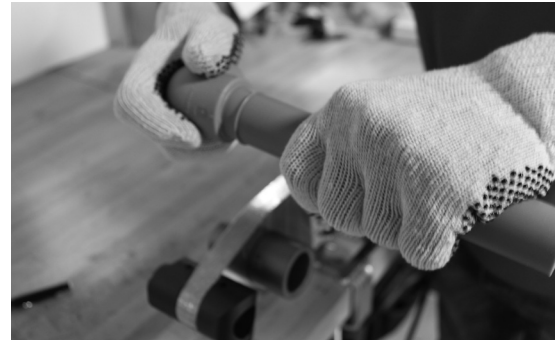
Figure F-4. Join fitting and pipe in the axial direction. During joining do not twist the pipe or fitting. Figures F-A, F-B, and F-C show the three welding process stages.
