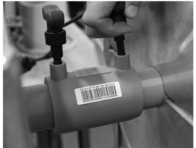
Figure F-20. Plug the cables in to the terminals of the electrofusion coupling.
