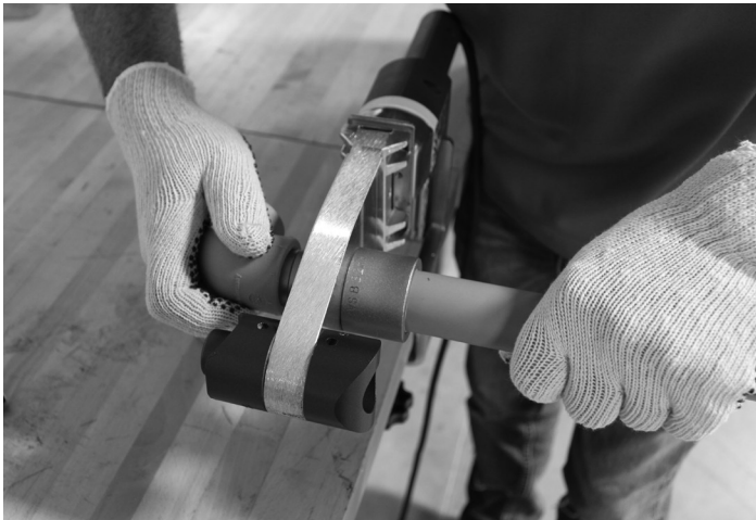
Figure F-3. Push the pipe end and the fitting onto the heating element of the hand socket welder in the axial direction. Heat pipe and fitting simultaneously.
