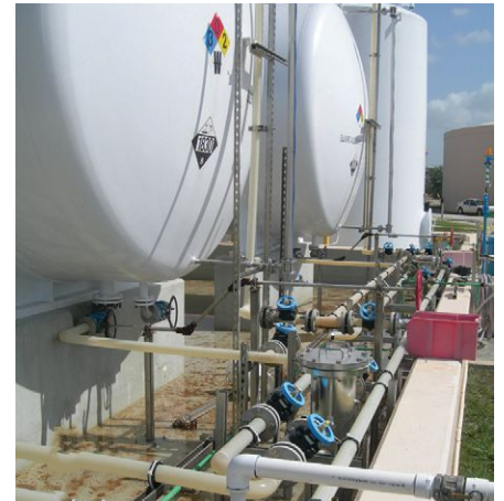
When utilized in a piping system, plastics create lighter and thinner piping while maintaining the necessary system pressure ratings.
